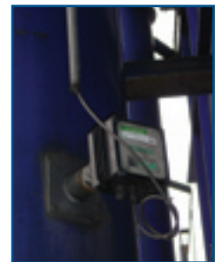
Electrodynamic Sensor installed in bag house outlet
