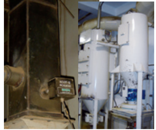
Cyclones on Drying Plant protected by fully insulated sensors
