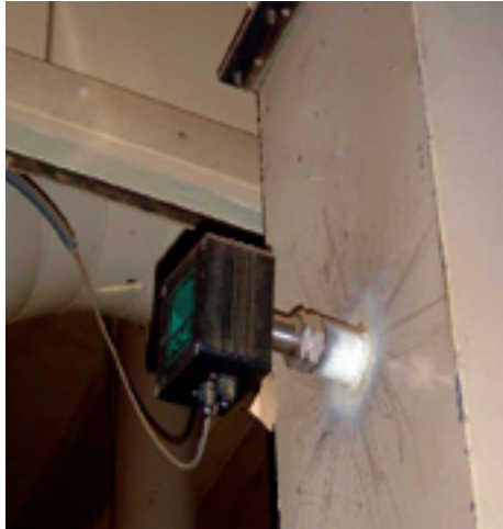
Part of a network of 18 sensors monitoring the performance of filtration systems plant-wide
